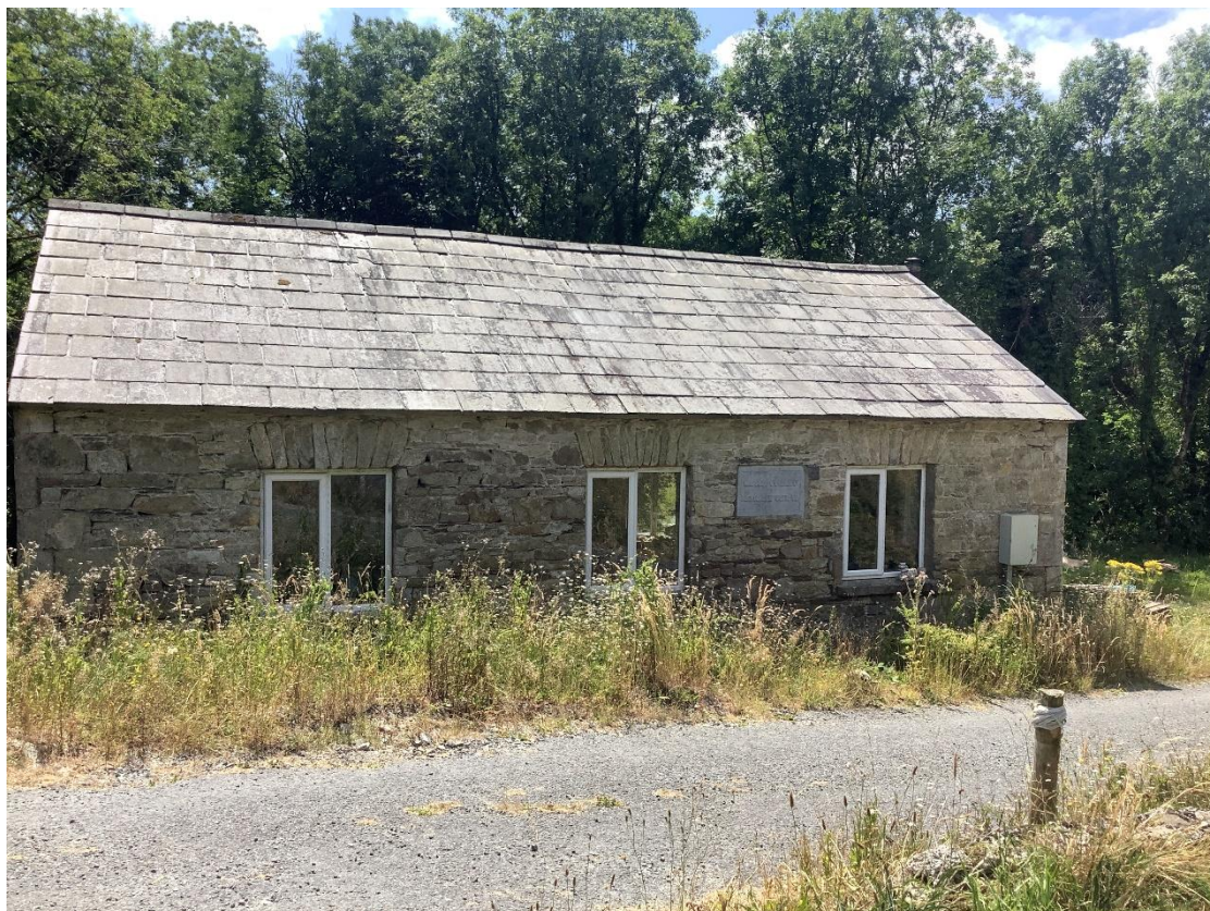
Plate 14-3: CH2 'Mountstuart School' adjacent to the Proposed 110kV Underground Cabling Route.
